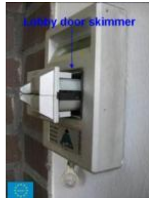
Figure 8: Image is Courtesy of EAST
